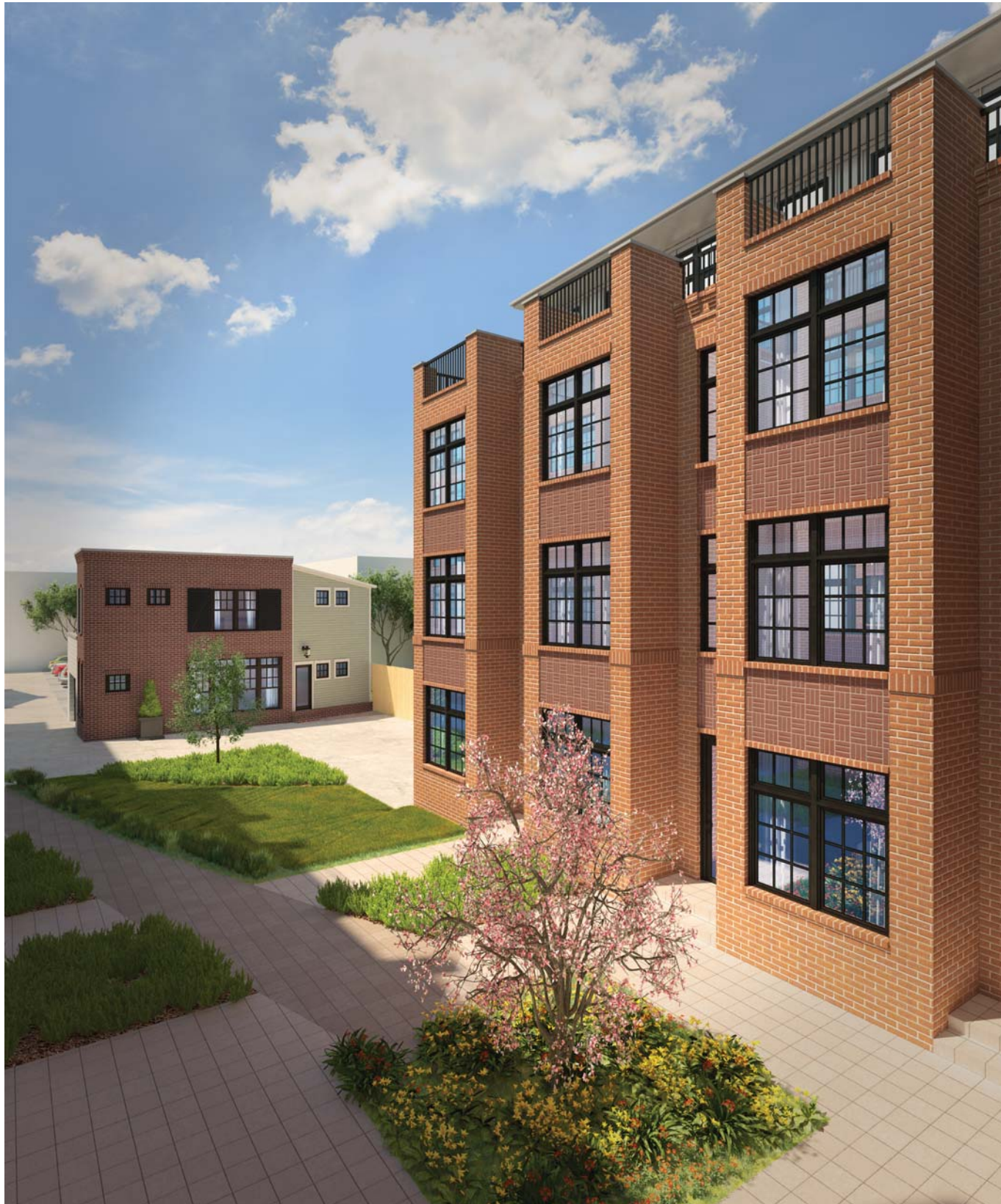
View looking South thru North Courtyard
