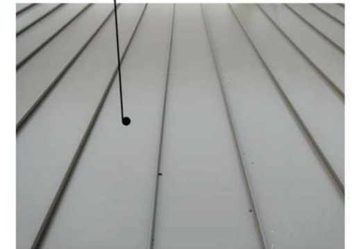
standing seam metal roof
