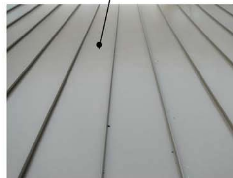
grey standing seam roof
