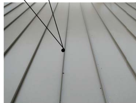
standing seam metal used as siding
